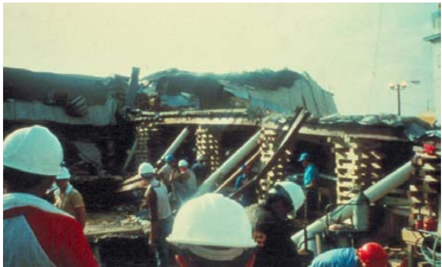
Figure 6:46 Sloped Floor Shoring
