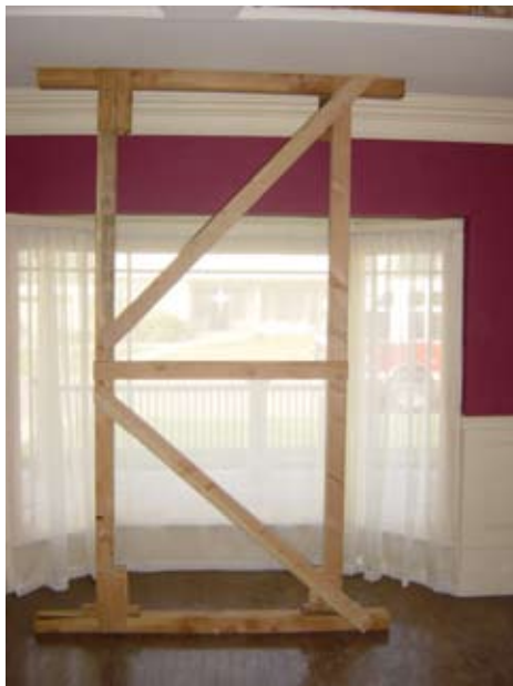
Figure 6:18 Two-post Vertical Shore (Class II)
