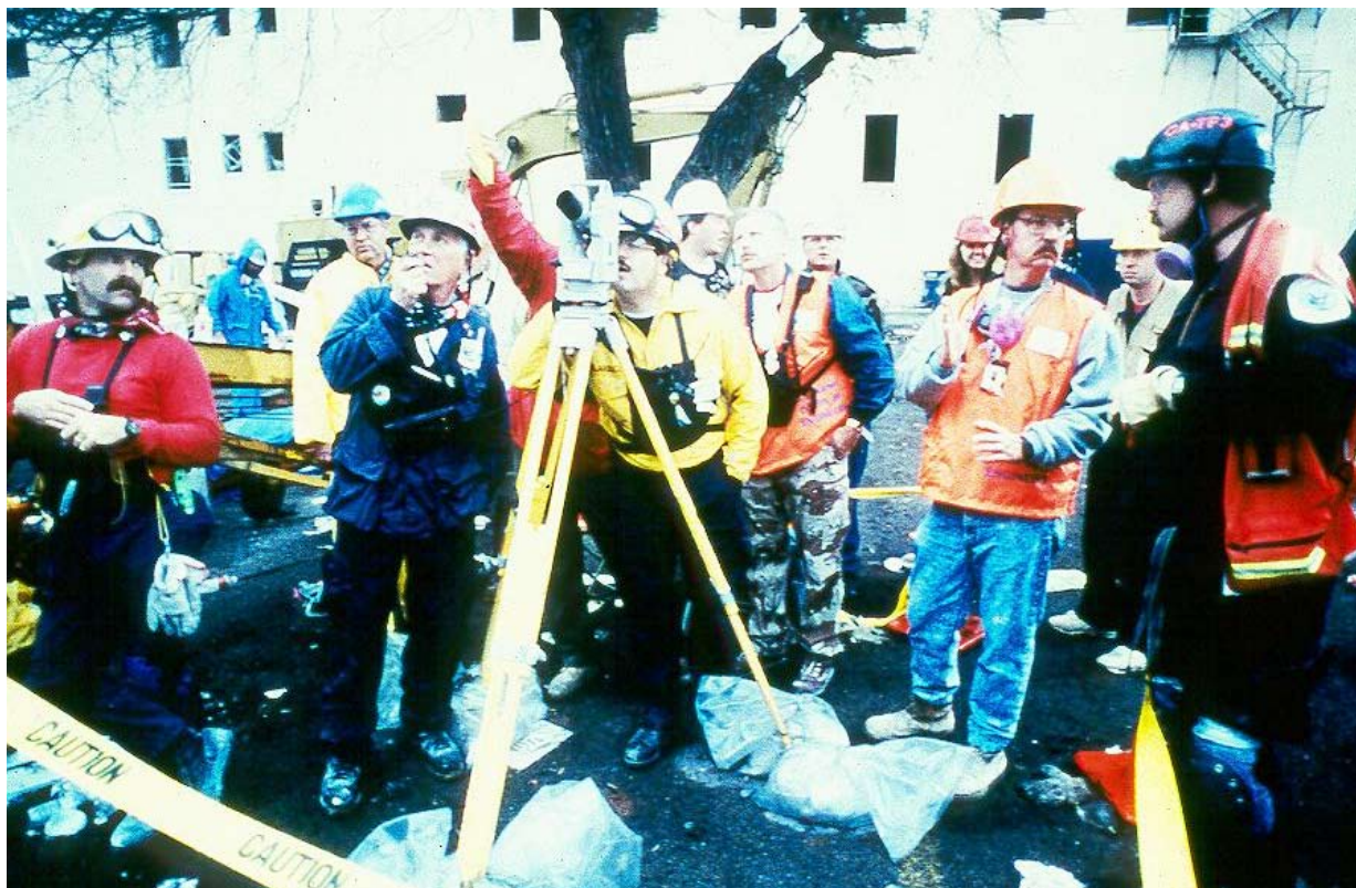
Figure 6:8 Monitoring a Collapse
