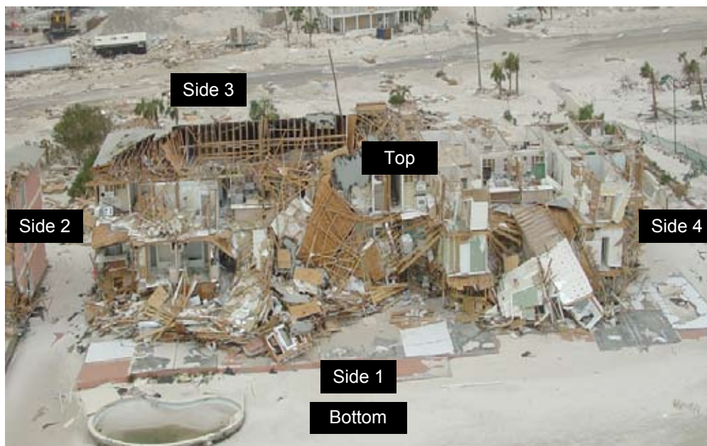
Figure 6:5 Sides of a Collapse
