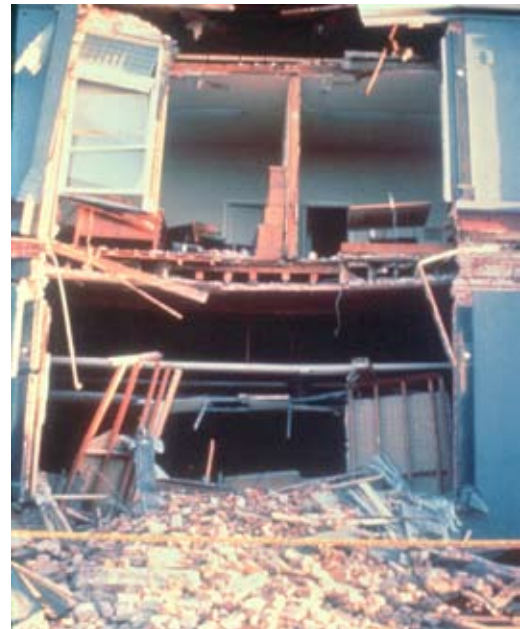
Figure 6:7 Unsupported Bearing Walls
