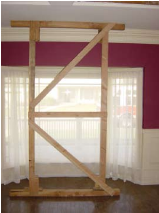
Figure 6.36 Two-post Vertical Shore
