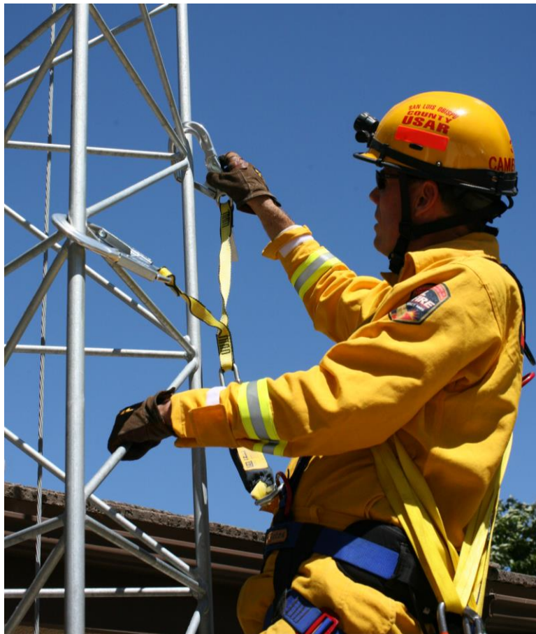
Figure 14-9. Rescuer protected climbing with bypass lanyard
