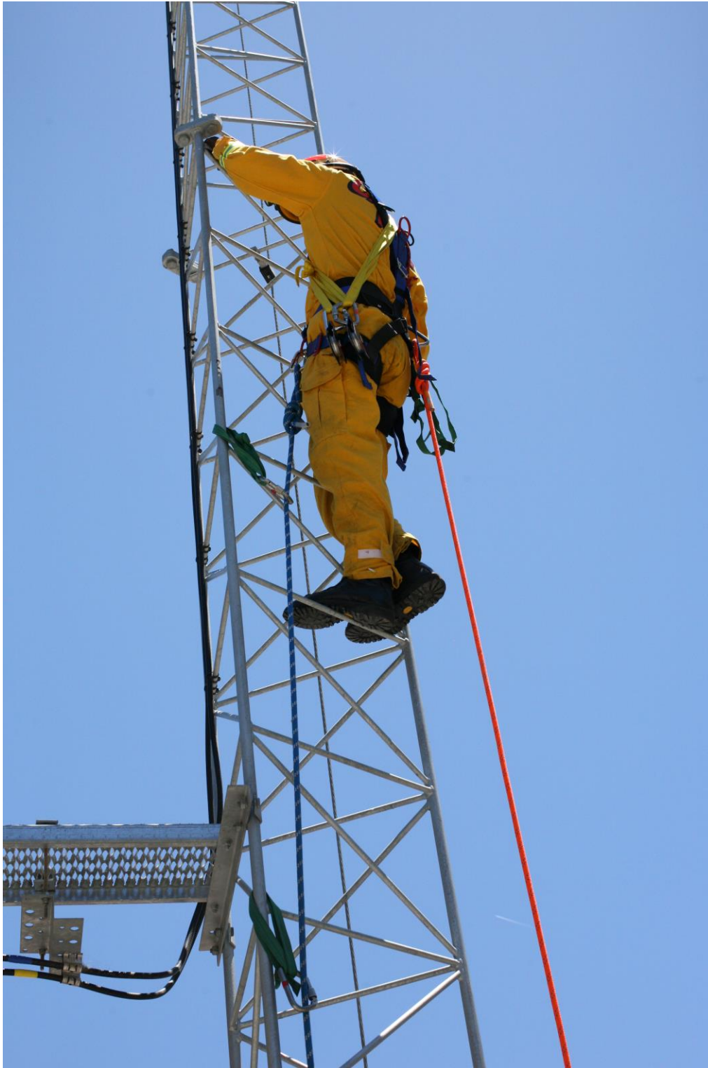
Figure 14-7d. Rescuer mid-way up protected climbing with a bottom belay (trailing main).
