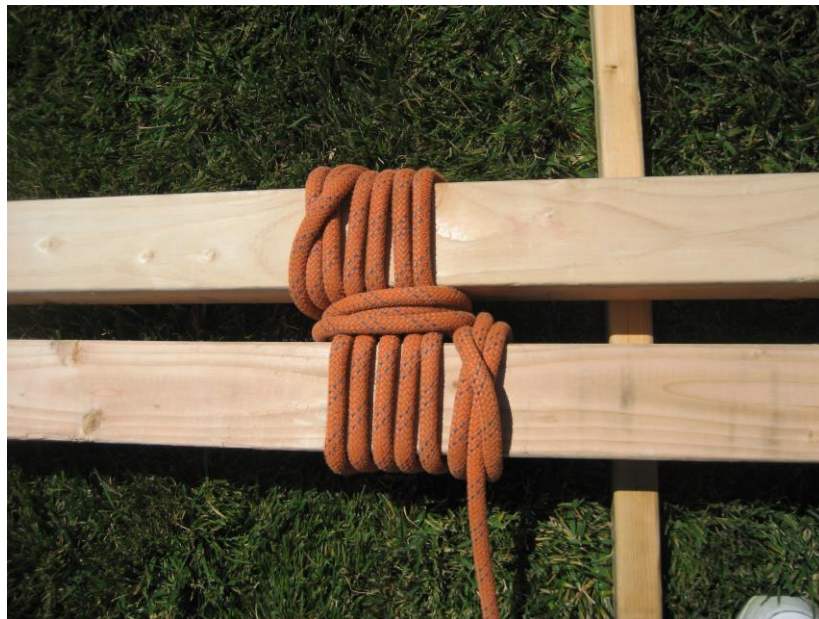
Figure 16-7. Secured with second clove hitch on opposite leg.
