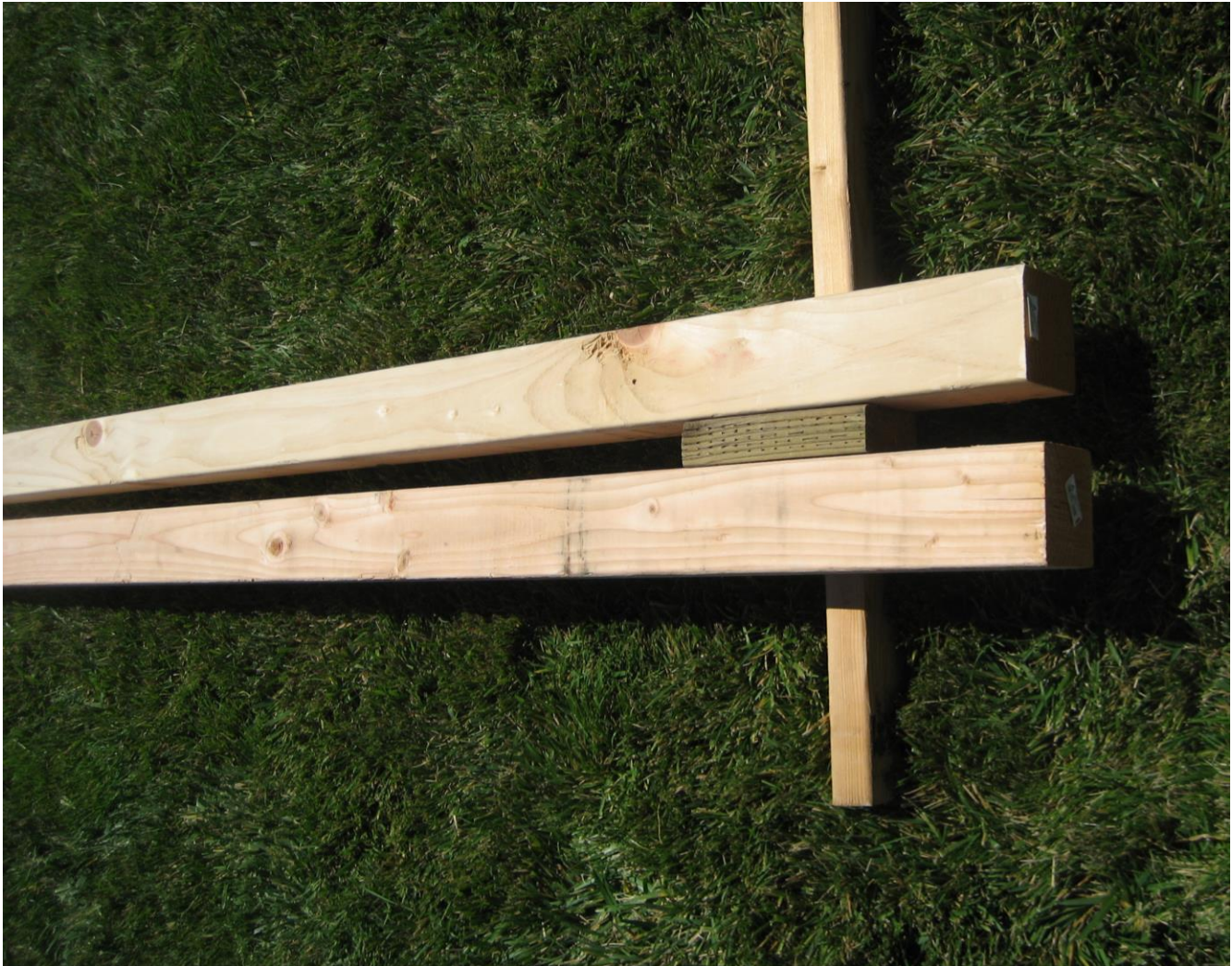
Figure 16-4. Starting an "A"-frame.
