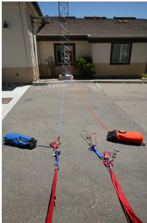
Figure 14-7a. Protected climb rigging with a bottom belay and main (for lowering).
