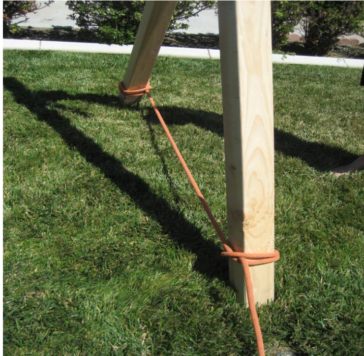
Figure 16-9. Hobble on legs of “A” frame.
